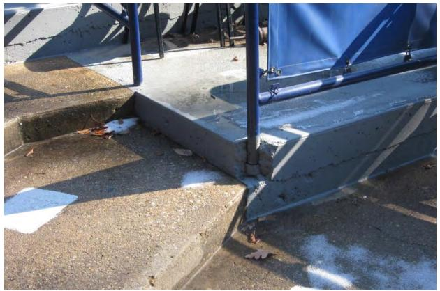
Characteristic concrete deterioration at Pavilion seating base, east side.
