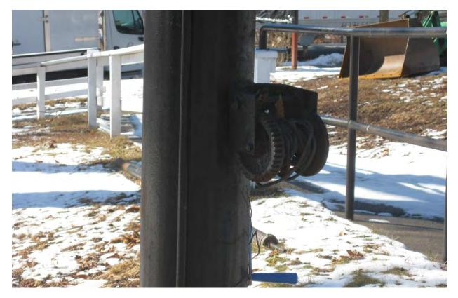
Failing winch hardware at Loge tent masts has required replacement as needed.
