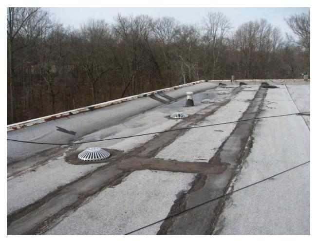
View of Pavilion roof above rear of stage. Roof, flashings and drains are now in need of replacement.
