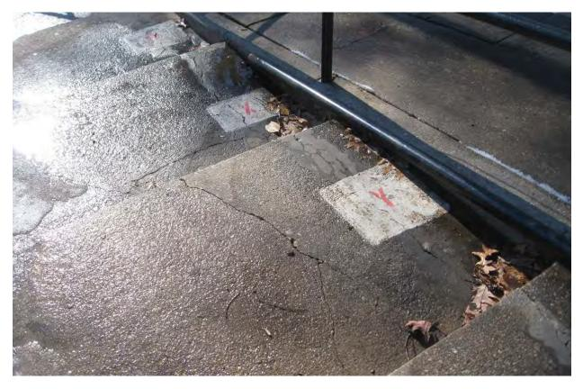
Characteristic settlement cracking East Loge seating base.
