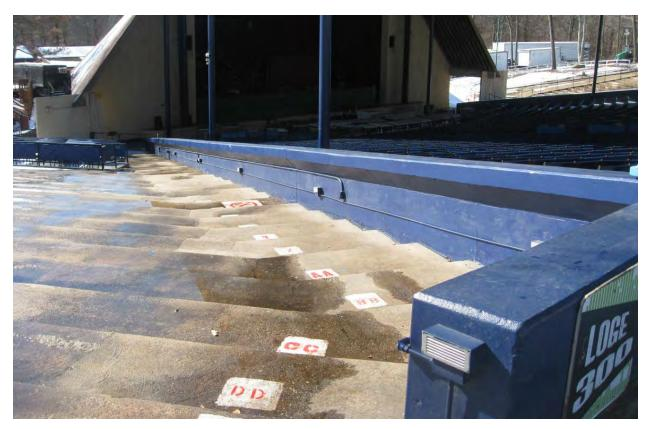
Original concrete cheek wall between original and newer Loge seating obstructs ingress/egress.
